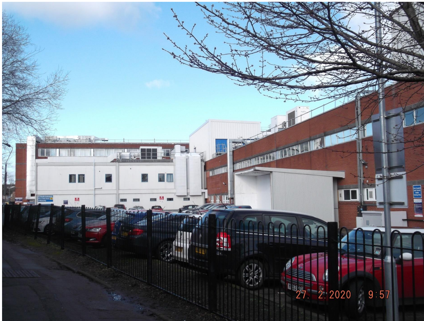
Site from Bridge Lane (2)
